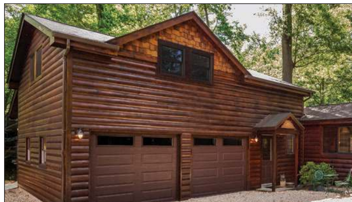
By raising the roof above the garage studio six feet (right) and adding windows, the remodeler freed up 770 square feet of floor space which is now used to support two art studios and storage space. The Thorntons use their independent work rooms several times a week. Chris Arnold, a Foster partner, found matching logs for the second-level "pop-up" by researching available options with a variety of vendors.
